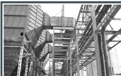
ESP for NTPC's Rihand Super Thermal Power Project
