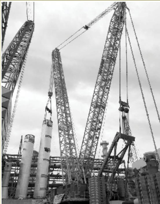
CO 2 ADSORBER column 51 mtr height and 550 MT weight being erected with 1600 MT cap main crane and 600 MT trailing crane at RFCL Ramagundam
