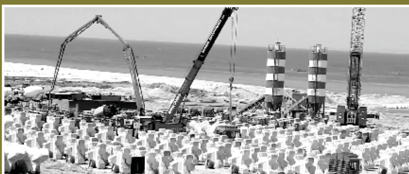
Casting and Staking of Accoropodes-II for break water development of Vizhinjam Port at Kerala for Adani Group
