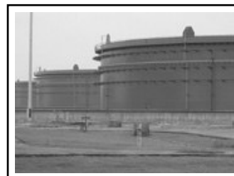
Double Deck Floating Roof Tank, 79 Mtr. Dia. X 13.5 Mtr. Ht. at IOCL, Mundra
