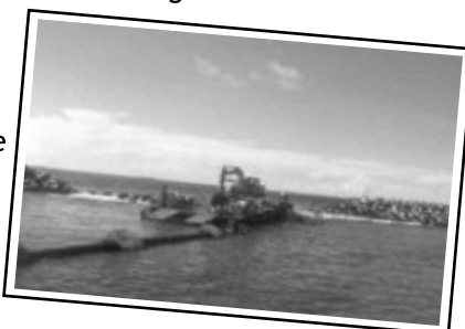
Work in Progress at Open Sea for Sea Water Intake Pipeline for Power Plant of State Electric Co., Maldives
