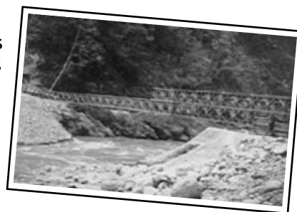
Launching of 180 ft. Span Bailey Type Unit Bridge over river Sutlej for Naptha Jhakri Power Corporation, HP.
