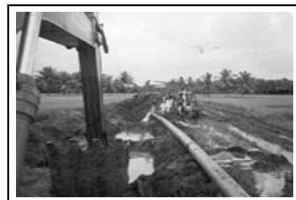
ROW & Welded pipes for cross country pipe line project at GAIL/KG Basin, Phase - II
