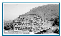
200ft span Bailey Type Unit Bridge at Rayagada for Govt. of Odisha
