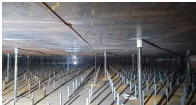
Lifting of Double Deck Roof of Floating Roof Tank by Jacking method in place of using water during construction.
