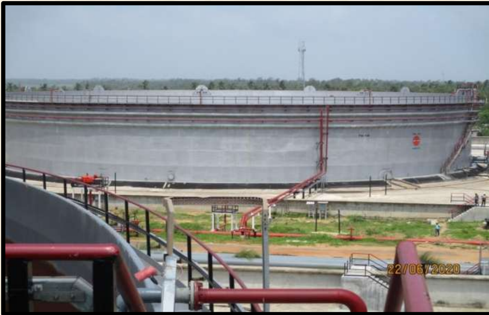
Turnkey Construction of 79 M Dia Double Deck Floating Roofs at IOCL Paradip Refinery
