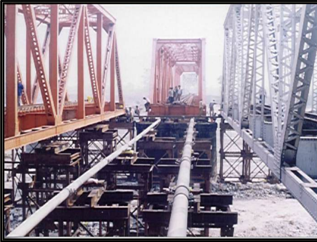
Regirdering of 7 spans X 45.70 metre each of Diana Bridge for Northeast Frontier Railway
