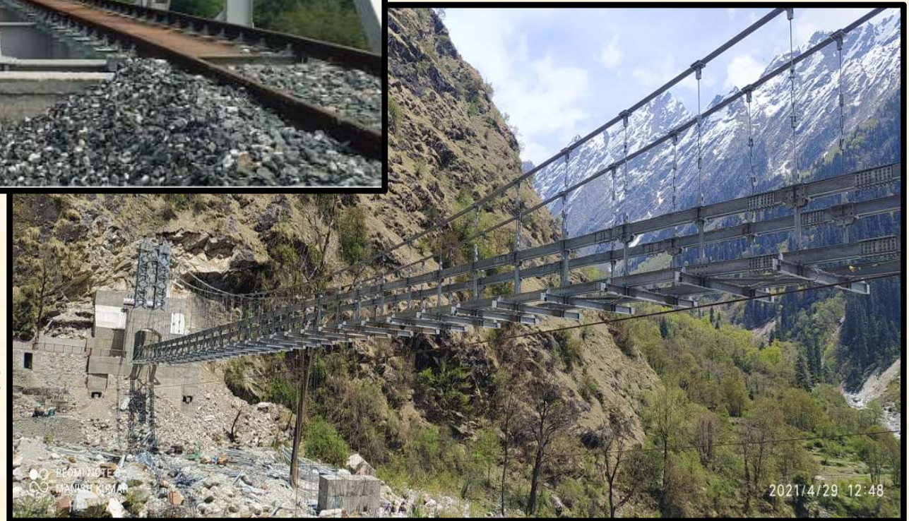
135 Mtr span Suspension Pedestrian Steel Bridge on Govindghat to Ghangharia Road at KM 10 in Chamoli District for PWD, Uttarakhand
