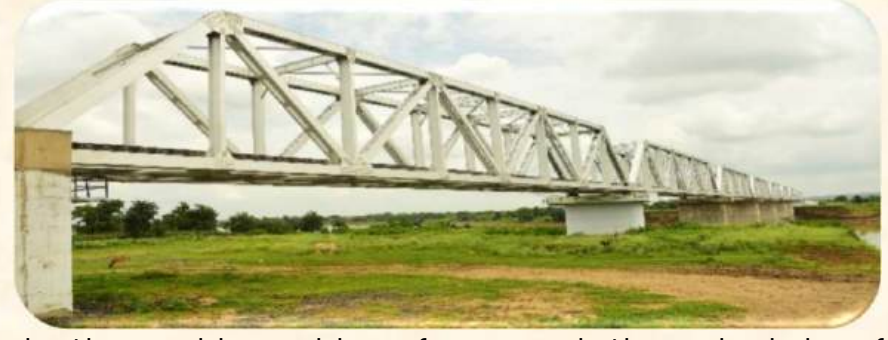
Fabrication and Launching of open web through girders for major bridges between Jhalawar-Aklara section for W.C.
