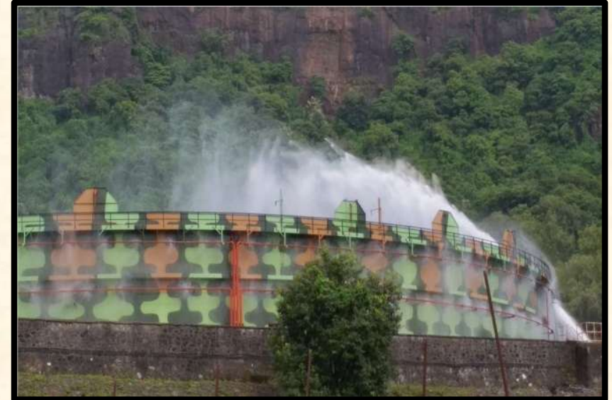
Fire fighting system for Crude Oil Storage Tanks at ONGC, Uran.
