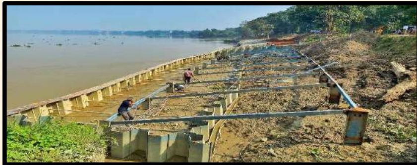
Sheet Pile & ISMB Driving
