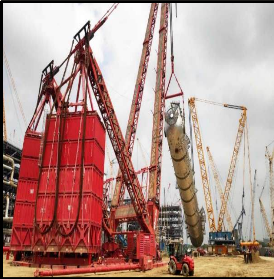
Erection of 1370 MT Equipment by 3200 MT crane and 1600 MT trailing crane at Bathinda Refinery of HPCL-Mittal Energy Ltd.
