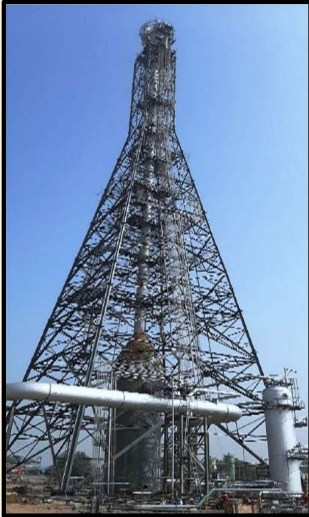
Flare Stack Structure - 135 Mtr. height at BS VI at Gujarat Refinery_vadodara
