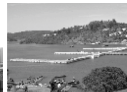
Piling & Marine Work
