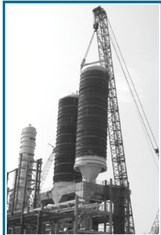
Erection of two nos. Coke Drums of 575 Mt each at CPCL, Chennai
