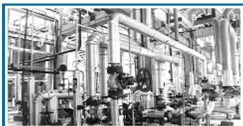
Piping Work at LLDPE of IOCL, Panipat
