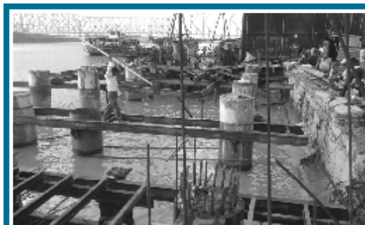
Hooghly River Front Development Work for Kolkata Municipal Corporation
