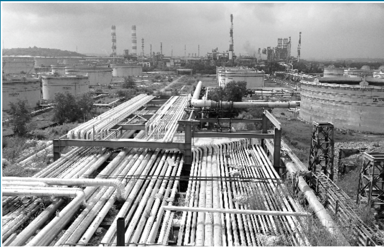
Tankage work and Offsite Piping at MRPL, Mangalore
