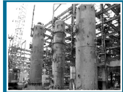
DCU Unit at BPCL, Kochi
