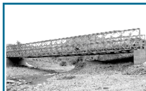
Bailey Type Unit Bridge at various locations for Govt. of Odisha
